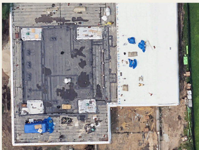
9.4 Existing roof, Clarendon Park Community Center, Chicago
